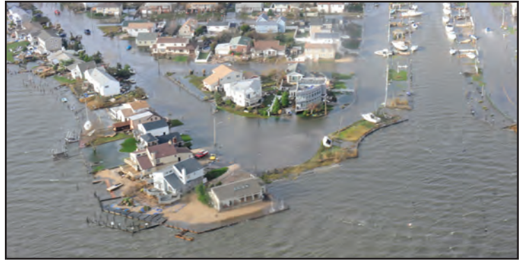
Aerial view of the flooding and structural damage caused by Hurricane Sandy in 2012. U.S. COAST GUARD PHOTO
